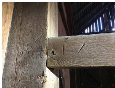
Figure 4.5 Mortise & Tenon Joint. A detailed interior view of a mortise and tenon joint within the Philip Pry Barn. Courtesy of Scott C. Woodard, US Army Medical Department Center of History and Heritage; November 2017.
