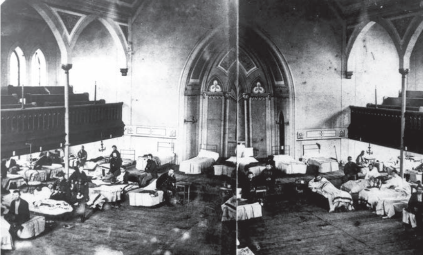
Figure 6.4 Lutheran Church—inside front. A composite of two photographs taken from the back of the sanctuary. This is the inside view of the Lutheran Church when it served as a hospital following the battles of South Mountain and Antietam. Source: Evangelical Lutheran Church, Frederick, MD. Accessed June, 15, 2020. https://www.twinspires.org/history
